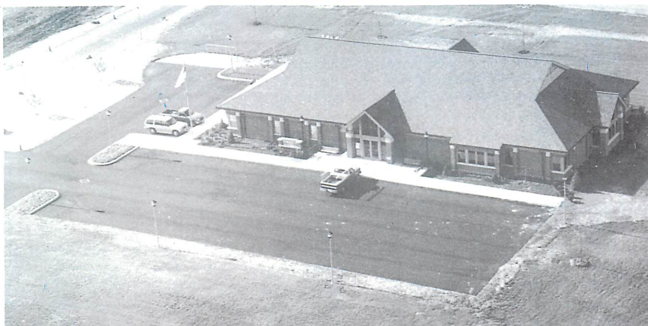
Aerial view of Fredericktown Library.
